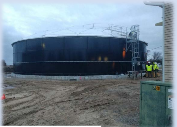
NEW 500,000 GALLON STORAGE TANK AT WILLIAMS TOWNSHIP PUMP STATION
